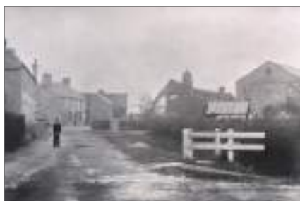
Water pump (right), the newly-built Baptist Chapel (distant right). The fire station shed (front left), the bakehouse (mid-left, with the two chimneys) and Lion and Lamb (distant left)
